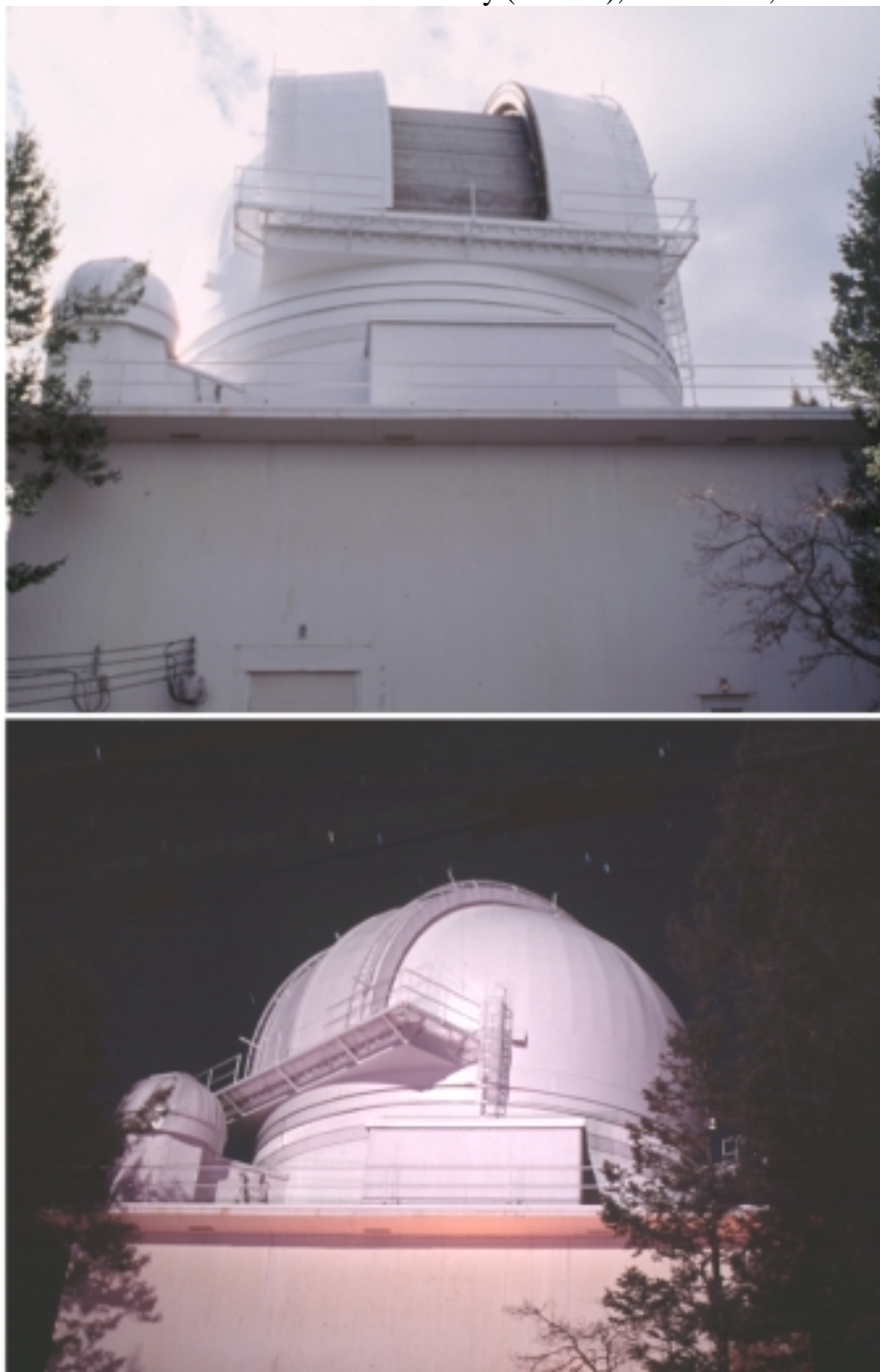
Figure P-3. Day and night views of southeast face of the NASA Orbital Debris Observatory (NODO). The upper image shows the 4.5m wide hemispherical slit of the 14.5m diameter main dome in the fully extended position with the interior windscreen visible. The top of the high-bay door leading to the 1000 m 2 building interior is visible left of bottom center and the entry door is visible to the right. Both images show one of the two secondary domes at the building south corner.
