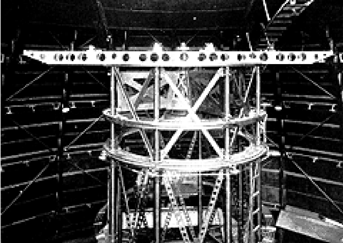
Figure 4.10. Original Michelson interferometer on the Mount Wilson 100-inch Hooker telescope.
