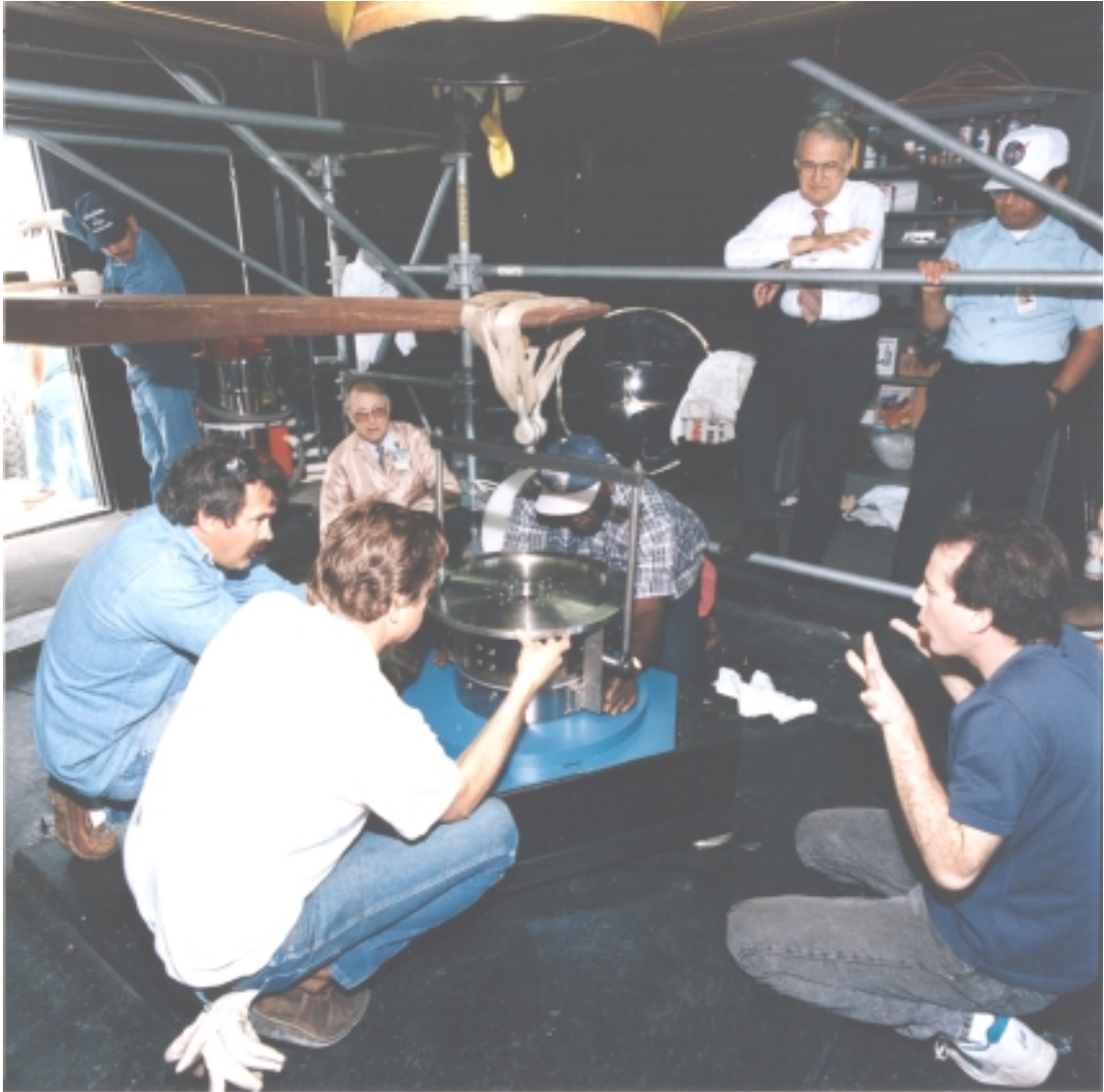
Figure II.B-21. View inside the NASA-JSC Silo showing the installation of the Professional Instruments (PICO) 10R Block-Head air bearing atop the I-Beam base. The bearing and direct drive motor were integrated into a 150 kg package. The bottom hub of the 3.0 meter mirror is visible at the top of the photo. The PICO air bearing enabled the LMT to become fully operational. Frank Gibbons is at left center facing the camera, Terry Byers is at right center, and the author is in the far right foreground.
