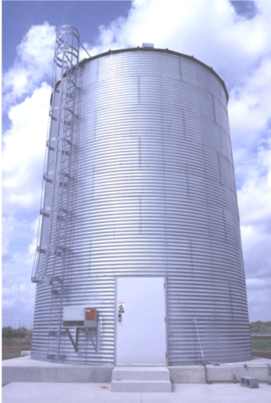
Figure II.B-13. Exterior view of the grain silo used as the testing facility for the NASA-LMT at the Johnson Space Center, Houston, TX. The 7.3 m diameter by 12.2 m tall structure had a removable 3.4 m diameter ceiling aperture which was covered with a removable polyethylene coated tarp. This cover was manually removed for nightly observations. The silo was sufficiently tall to provide the mirror with partial protection from exterior winds and enable interior access to the radius of curvature. The silo still remains at NASA-JSC where it is used for storage.
